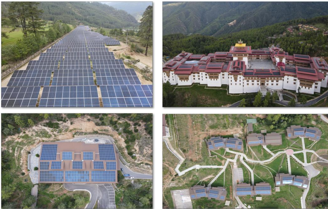
Figure 2. Phase II Solar Initiative Project (3.85 MW)
