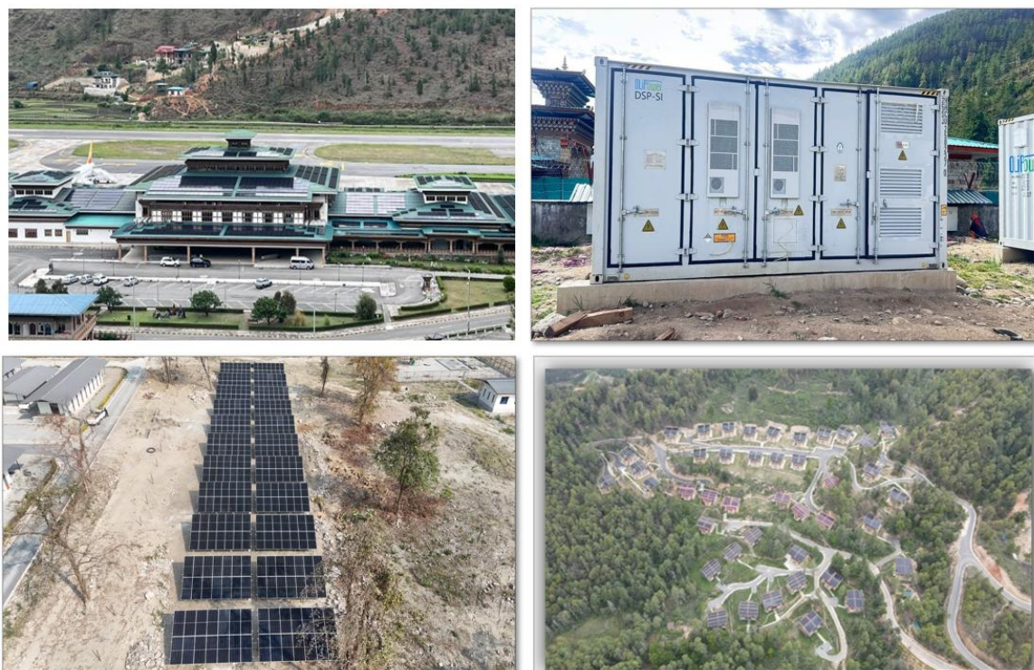
Figure 3. Phase III Solar Initiative Project (5.016 MW)
